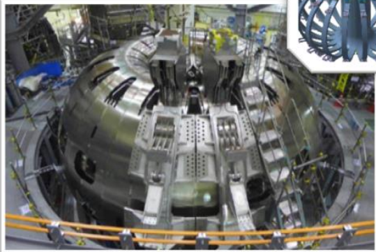
JT-60SA Toroidal Field Coil Casings
