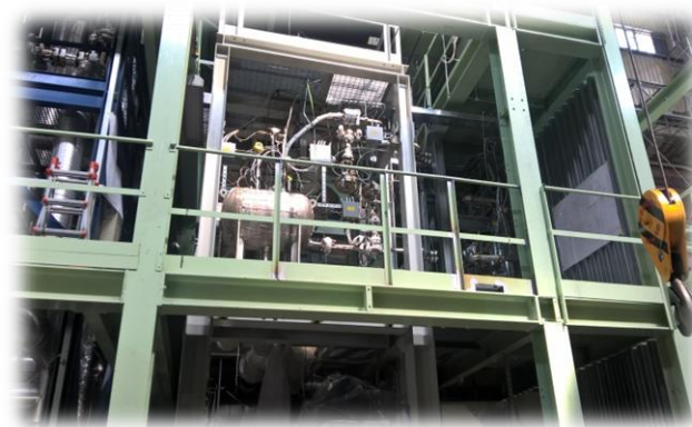
Test HAMmer in Lead Lithium (THALLIUM)
