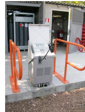
Dolomiti Energia Project: HCNG refueling station
